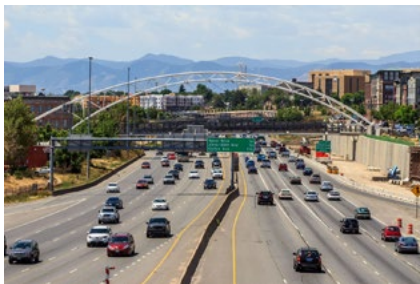
This $3 million project expands the lifespan of both bridges (Speer Boulevard Bridge shown here) and provides better clearance under the arch bridge girders on southbound I-25. Photo source: enverinfill.com
