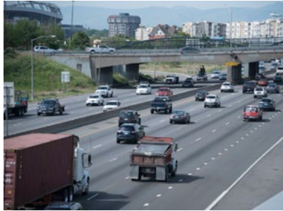
The 23rd Avenue Bridge, shown here, will be under construction for repair until this November. Photo source: hamoninfrastructure.com
