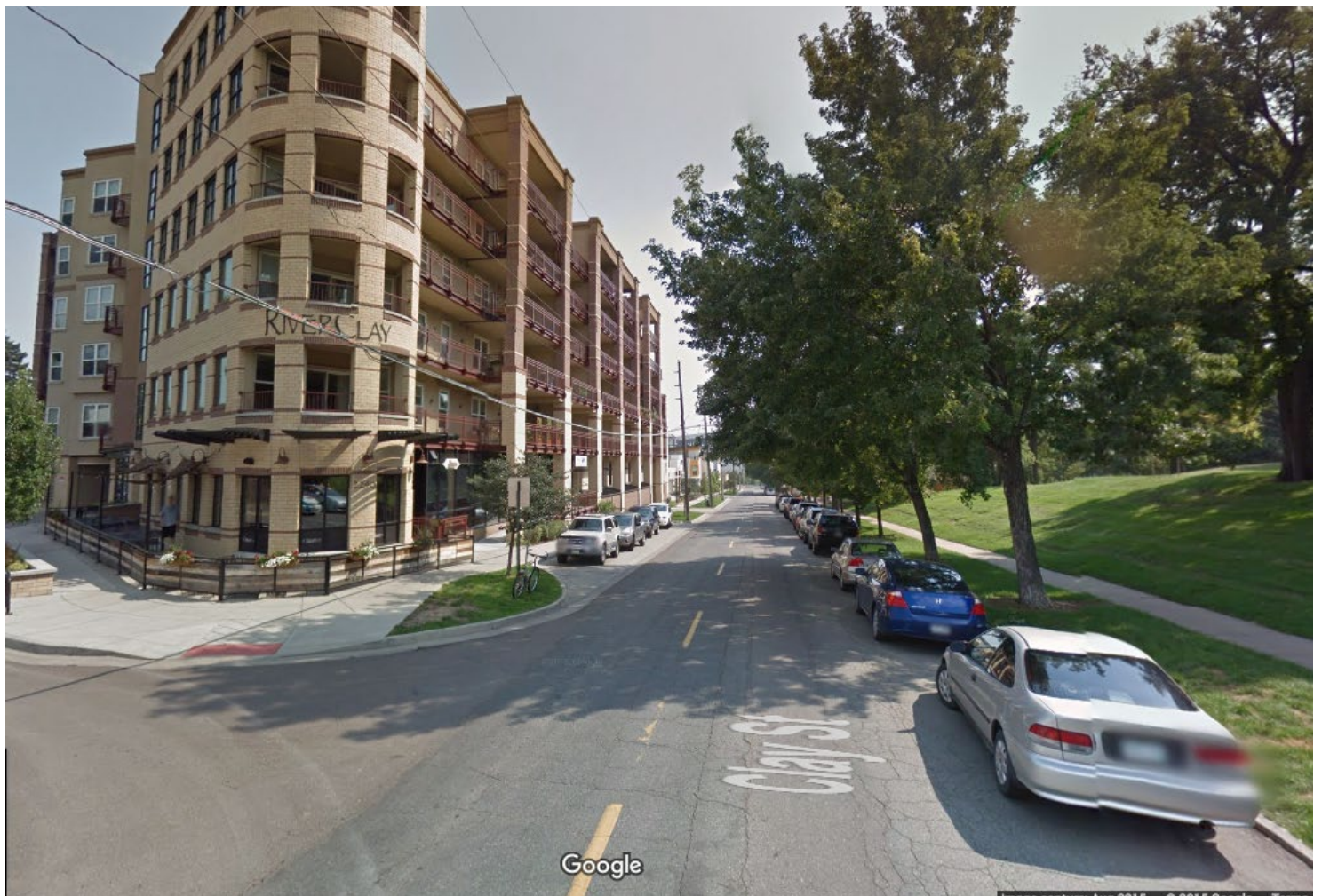
Google Street View of River Clay, looking towards the Stadium. Google Street View images belong to Google.
