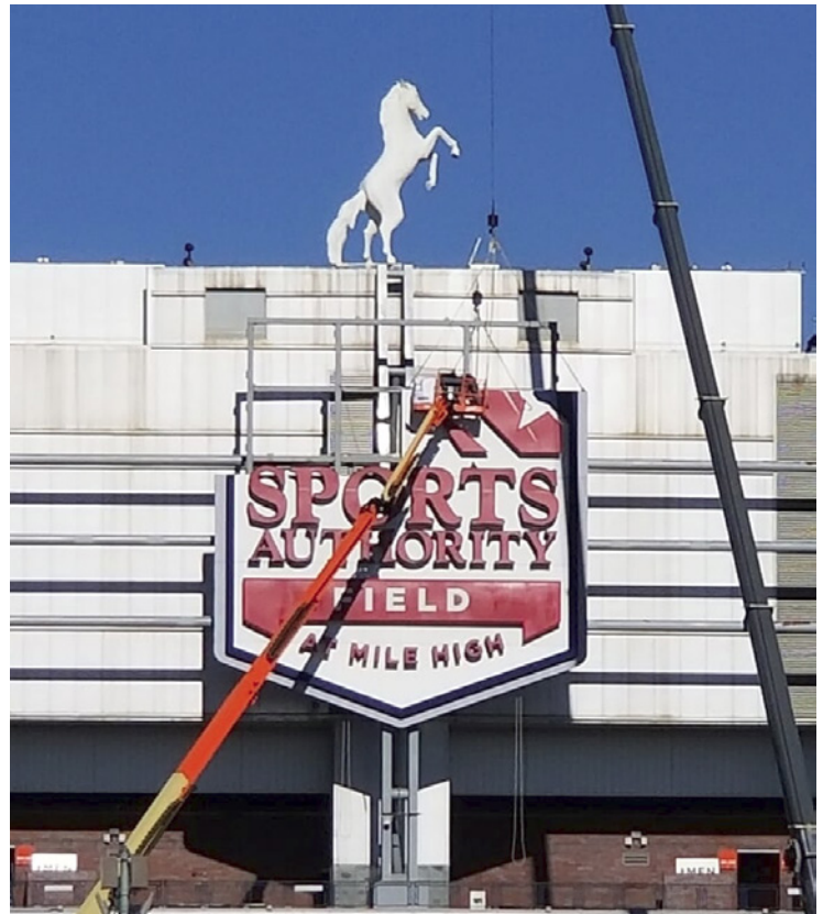
Removal of the Sports Authority Field at Mile High Signs
