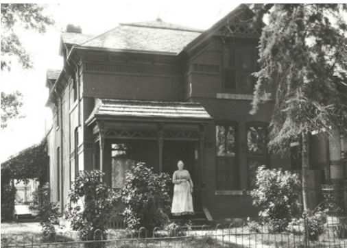
2550 River Drive. Built in 1886, this Victorian is one of about 18 homes on River Drive that could become Denver's newest historic district. Photo Courtesy of Denver Public Library
