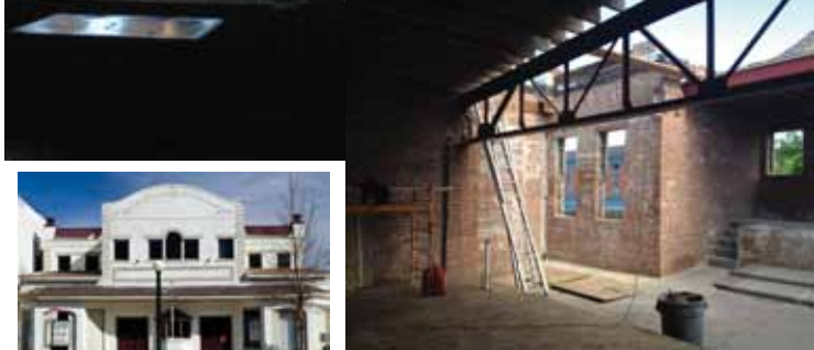
Construction Photos - Ryan Gruver
