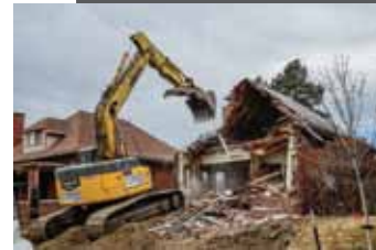
Making way for New construction 22nd & Elliot photo Jerry Olsen
