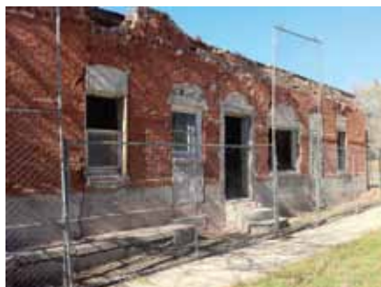
Old Gas Station Demolition Reveals History photo Jerry Olson
