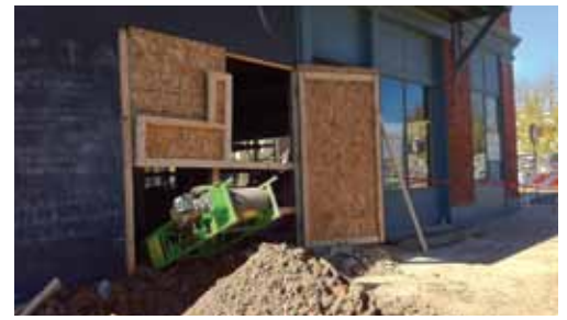
Basement Excavation at Sarto's see Jerry's article on page 4
