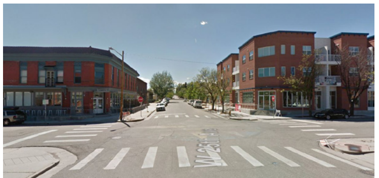
The corner of Eliot & 25th Street, looking west, 2017
