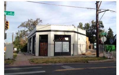
Construction happening at 23rd Avenue and Clay. Photo by Holley Petrick
